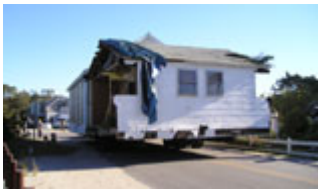
Rear view of the church being moved:
