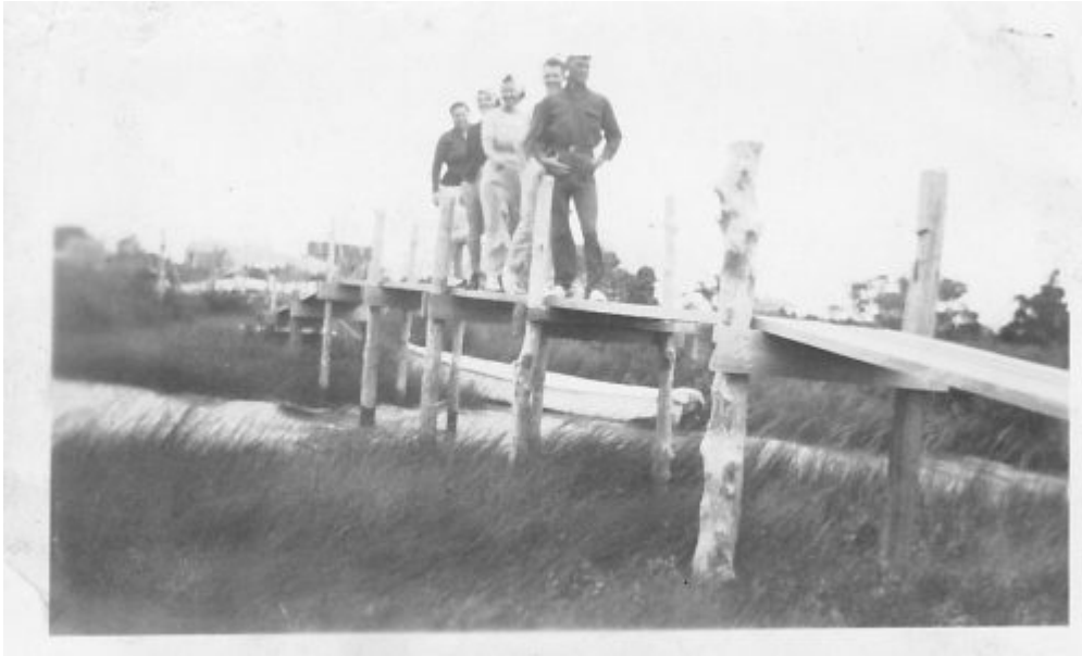
Bridge over gut
