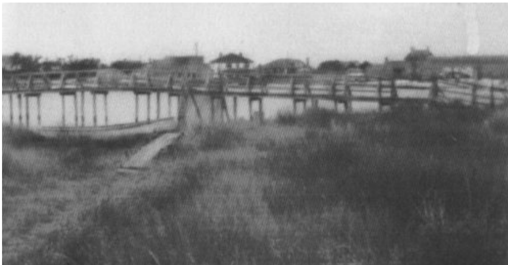
Bridge over the Gut
