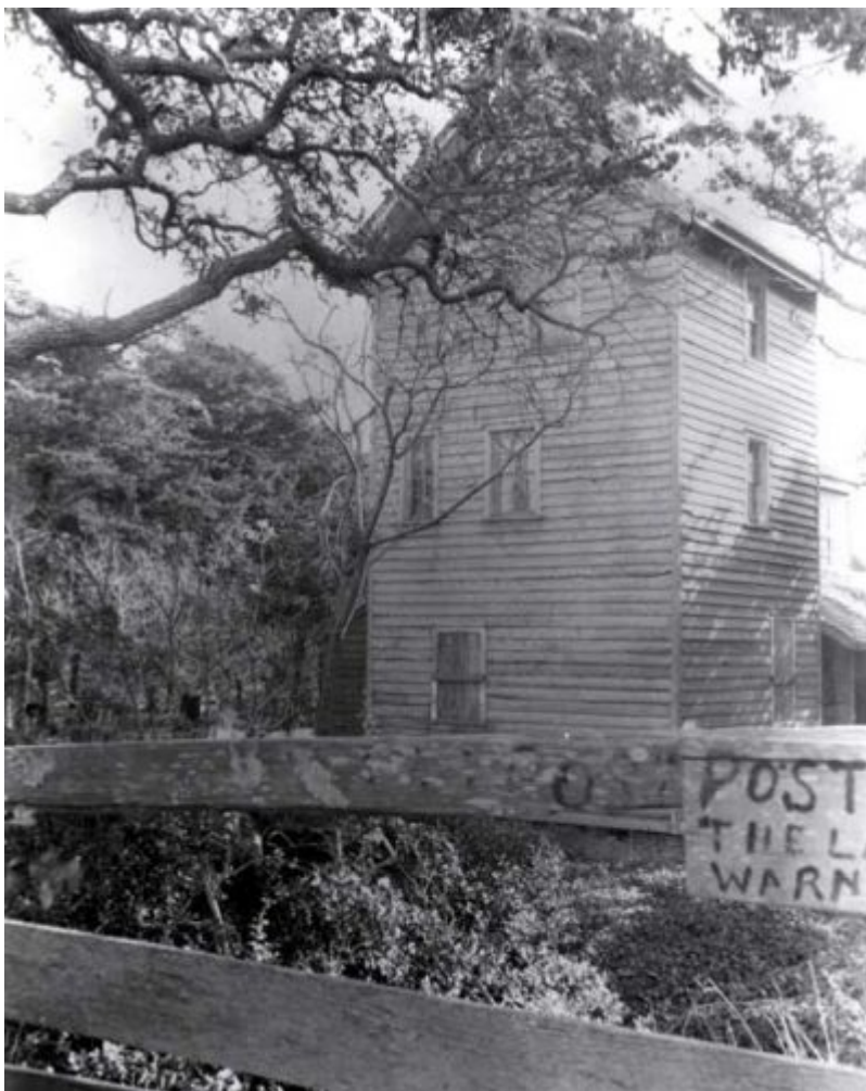
House at Springer's Point
