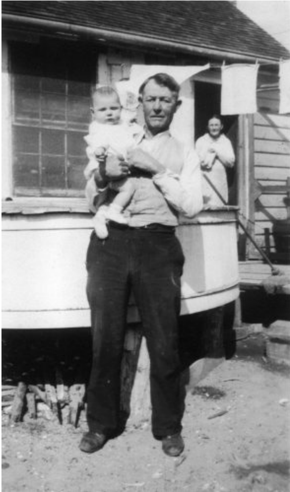
Ocracoke Conical-topped Cistern (dismantled in the 1970s):
