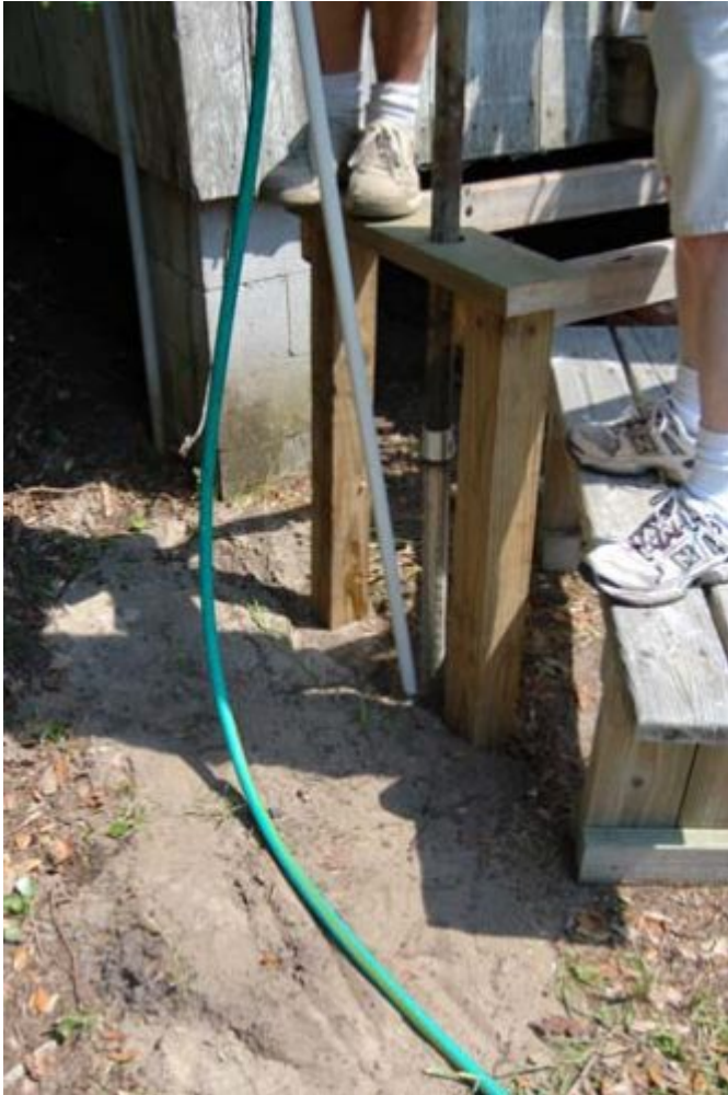
Working the Well Point Down:
