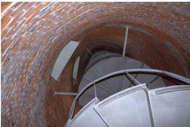
Ocracoke Lighthouse Spiral Staircase
